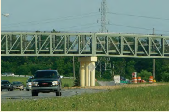
Photo of the newly completed Clinton River Trail bridge over Telegraph Road. Photo Source: m-bike.org
